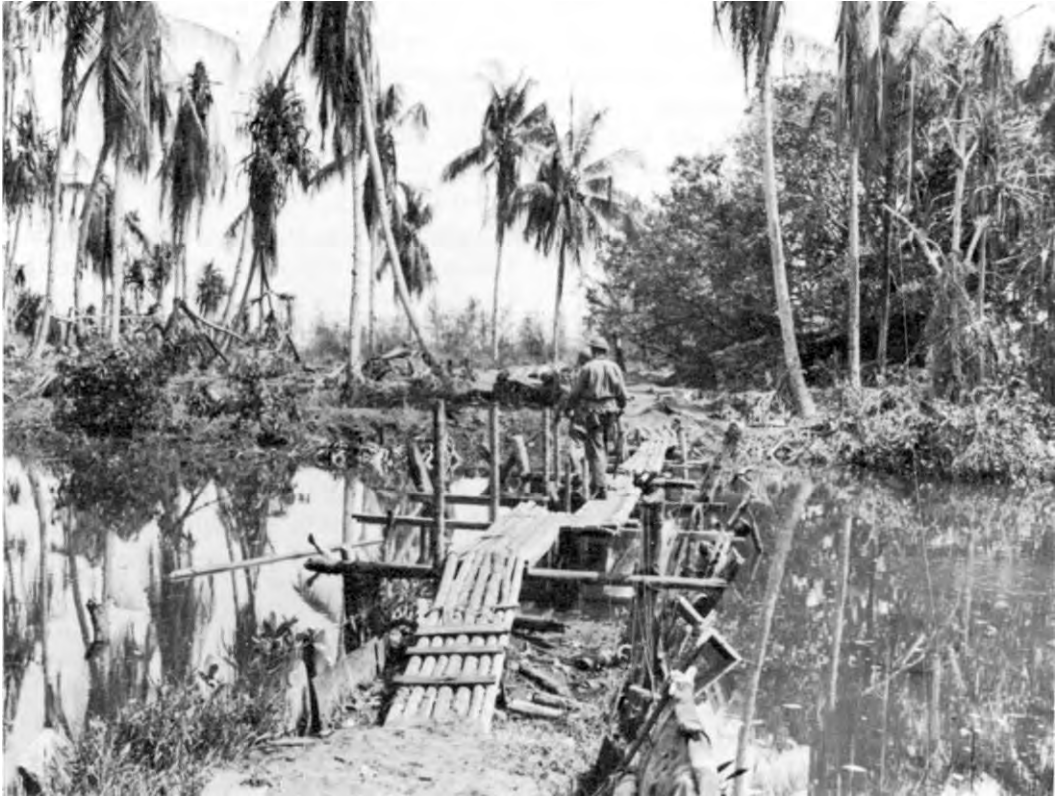
FOOTBRIDGE OVER ENTRANCE CREEK to Musita Island .
