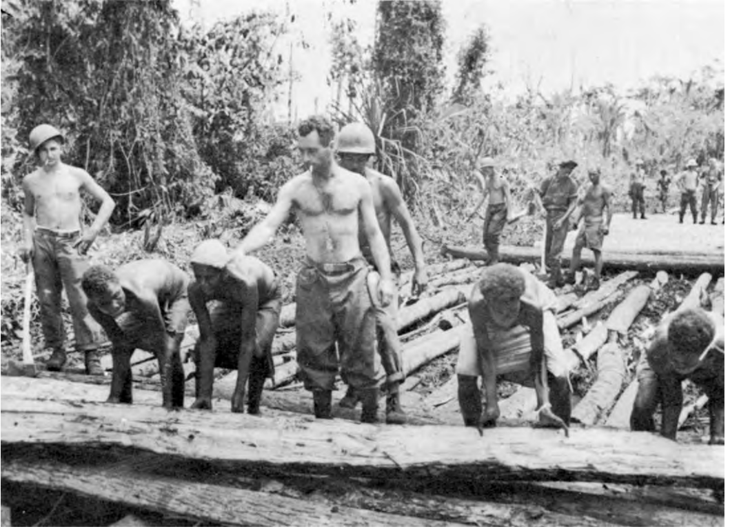
114TH ENGINEER BATTALION builds a corduroy road with the help of natives.
