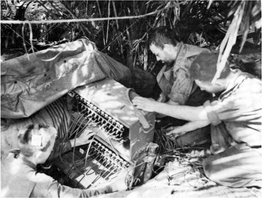
SETTING UP A FIELD SWITCHBOARD
