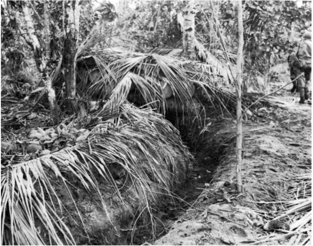
COCONUT LOG BUNKER WITH FIRE TRENCH ENTRANCE in the Buna Village area.
